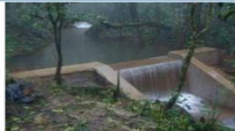
Construction of check dam.
